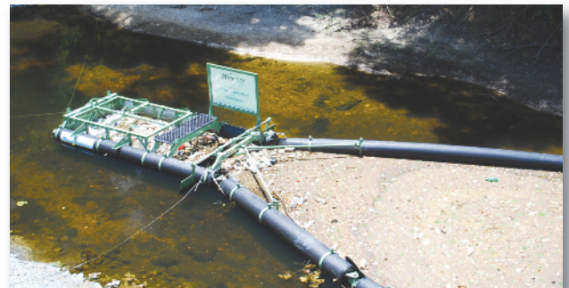
Bandalong Litter Traps, developed by Storm Water Systems, have been installed on the Satilla River near Waycross, the Anacostia River in Washington, D.C., and on the Arkansas River near the Clinton Presidential Library in Little Rock, Ark.
